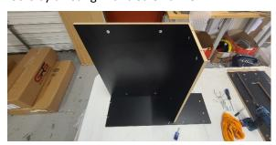
3. The next pieces to be installed is the bottom back panel and the top panel that holds your control panel. The bottom panel will be facing the back so make sure the cam locks are facing towards the inside. The top panel has predrilled holes for a back door clip. That clip should be facing towards the back of the unit. Lock into place as you go.
